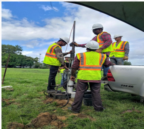
Figure 59: C.P.T. execution (soil quality inspection) by lab personnel
