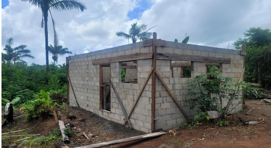
House construction Hinterland
