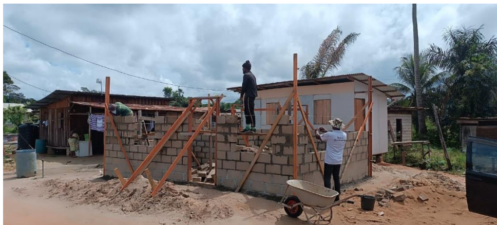
House construction Hinterland
