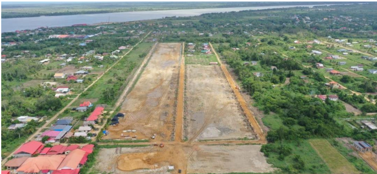
Civil works progress, Voorburg, Commewijne
