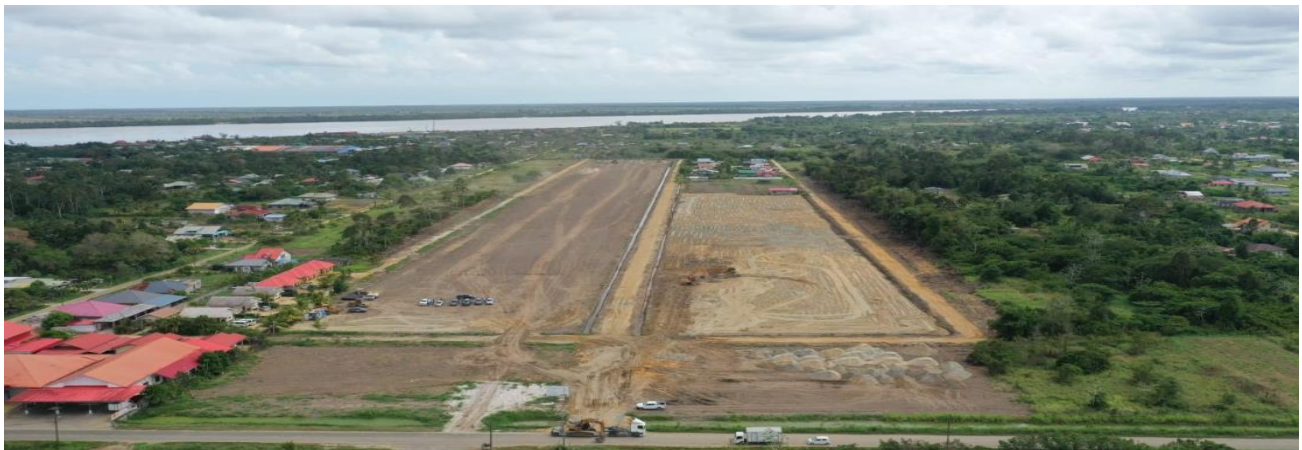
Civil works progress, Voorburg, Commewijne
