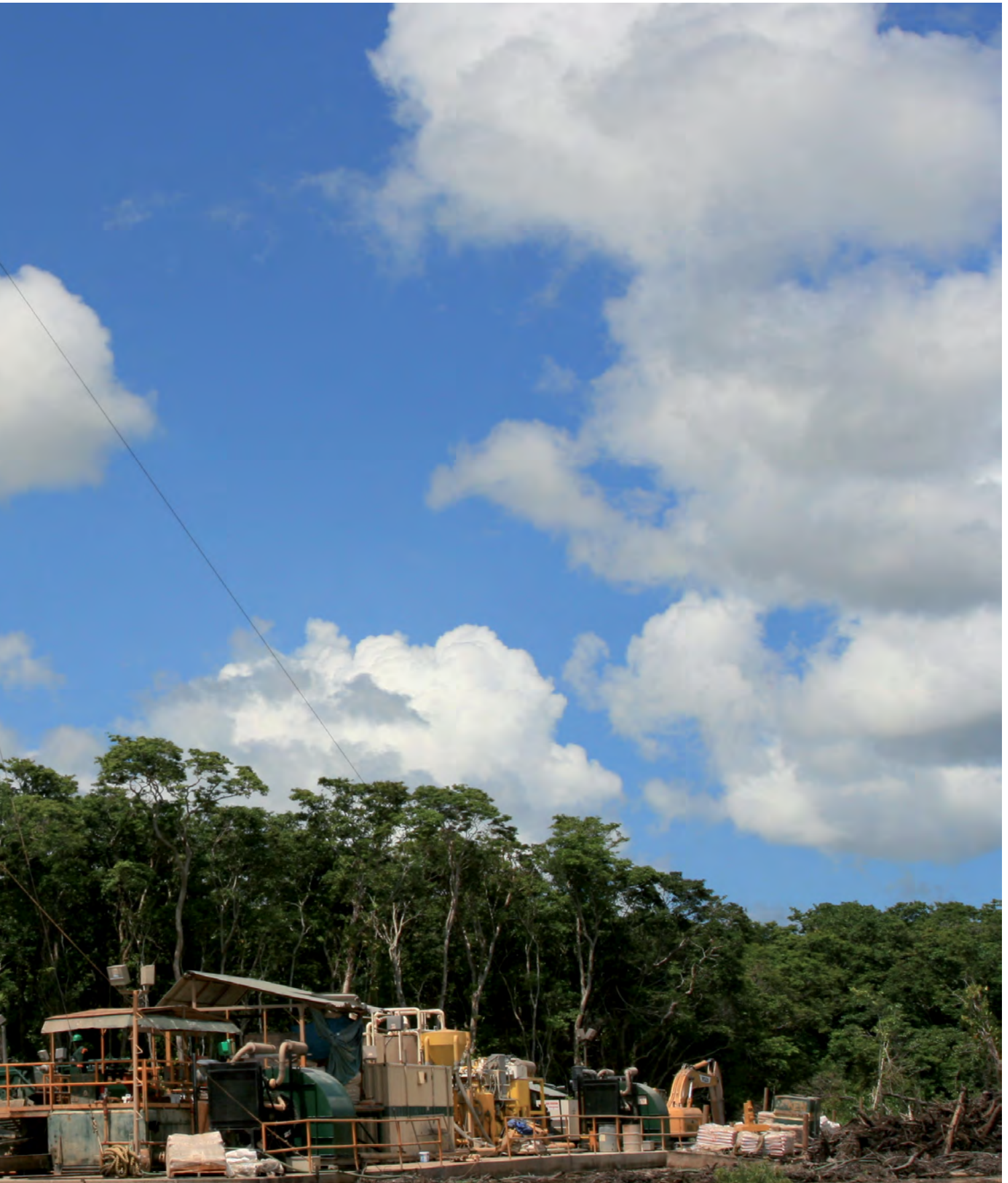
■ Production drilling in the Tambaredjo-Northwest oilfield.
